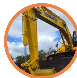
Slope Building in Pond
